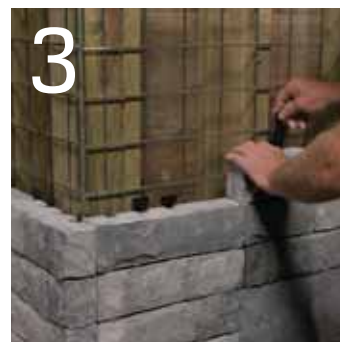
Attach Tandem Veneer with Connector
