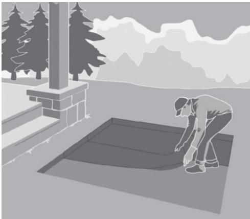
STEP 3: LAY GEOTEXTILE
