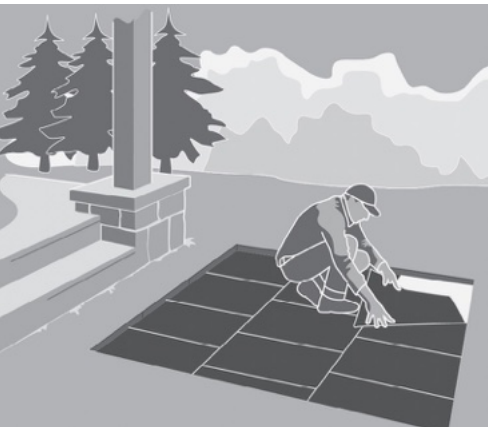
STEP 5: INSTALL EZ BASE PANELS
