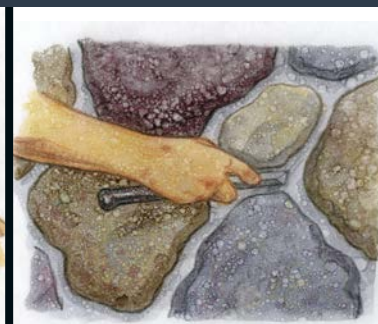
FINISH THE JOINTS
