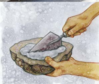
APPLY THE MORTAR
